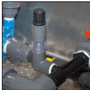
Mazzei® venturi air injection system (55-0126) sustains beneficial aerobic microbes while preventing bacteria from turning odorous and anaerobic
